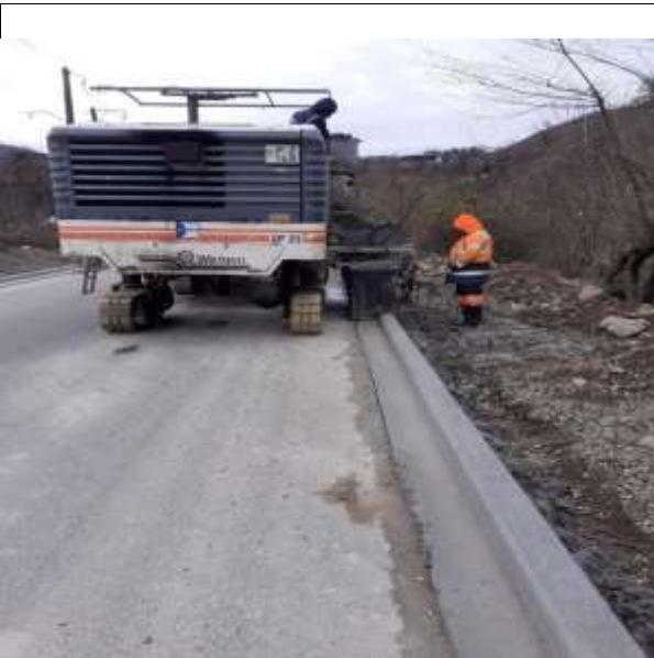
KM 2+460 – KM 2+590 (LHS) Casting Lean Concrete
