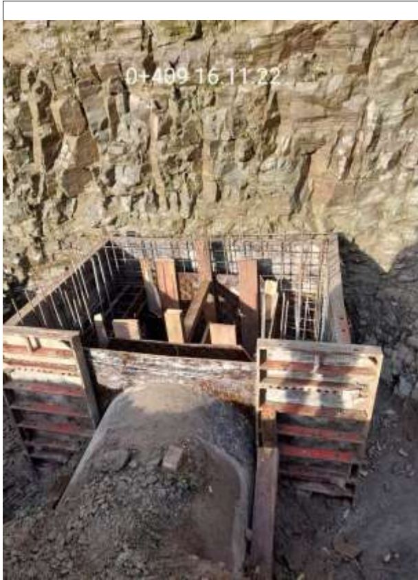
KM 0+409 Installation of Pipe
