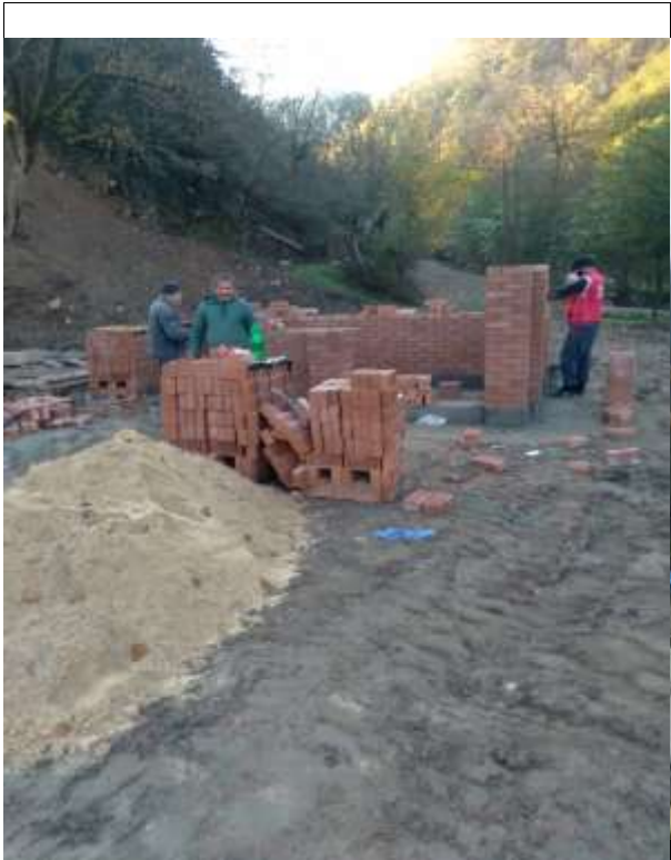
KM 2+467 Construction of Bus Stop
