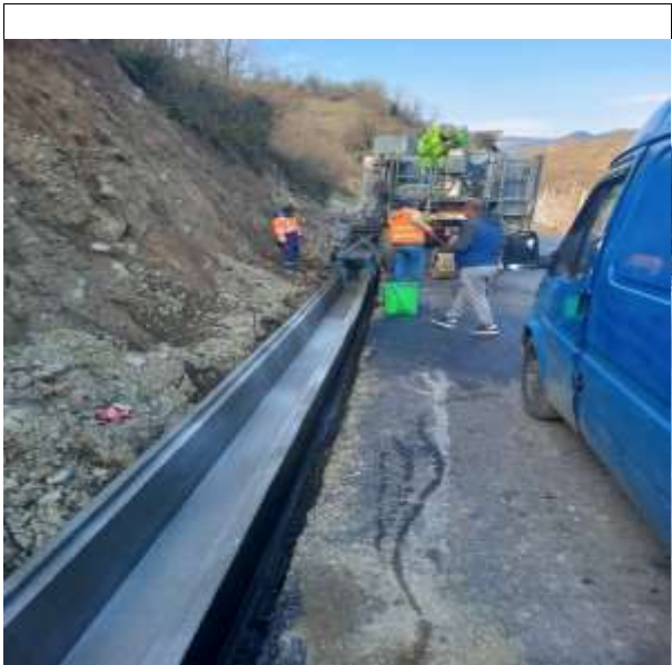
KM 6+550 – KM 6+750 (LHS) Casting Lean Concrete
