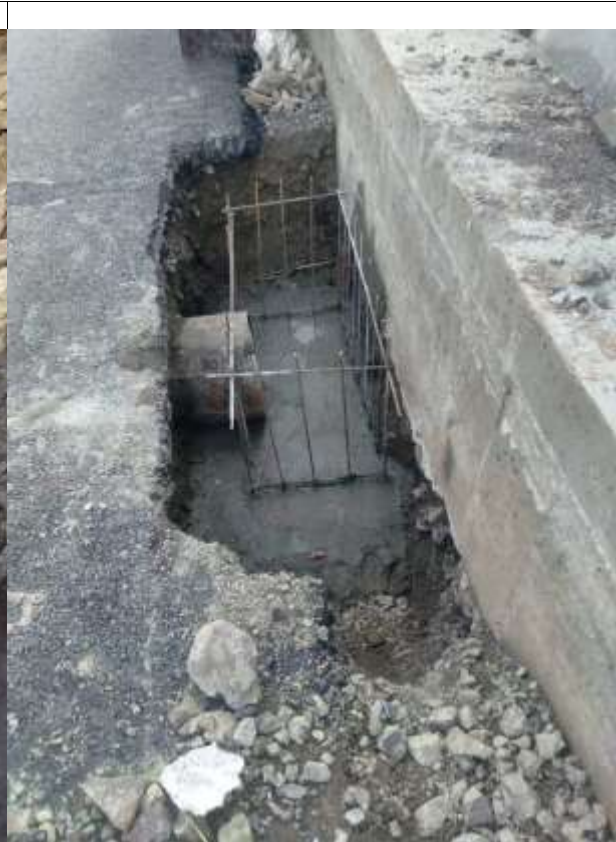
KM 6+428 Installation of Pipe.
