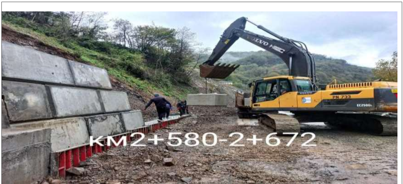
KM2+580–KM2+672InstallationofLego Blocks
