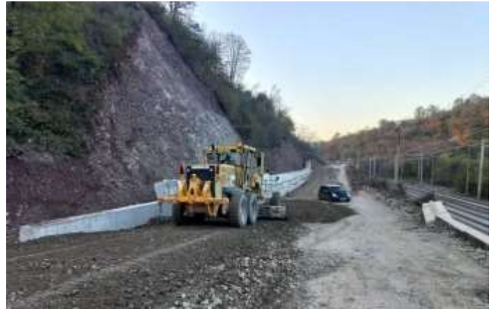
KM6+110– KM6+290Excavation, Cut, Fill.
