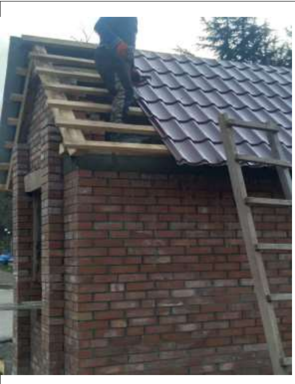
KM 14+822 Construction of Bus Stop
